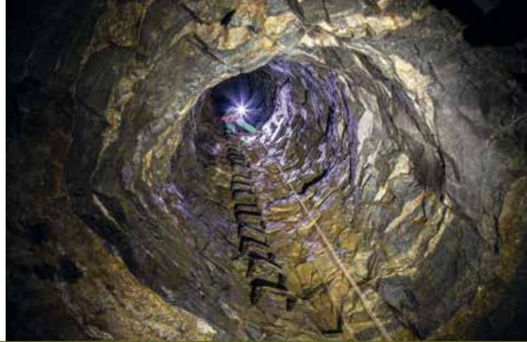
126. Left: Fonticelli mine, in Manoppello. Connection shaft between two levels of the mine with service ladder.
